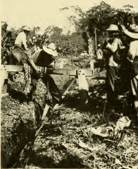
LOWERING PIPE INTO DITCH
